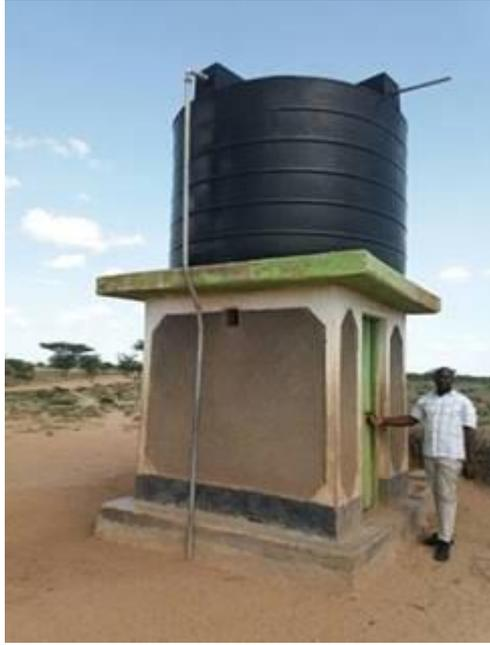
*Water storage facilities set up by Oxfam in Chok Chok are helping to build resilience in drought crises. These storage tanks hold up to 2 days of water supply to prevent water shortage in instances of water system breakdown.*
